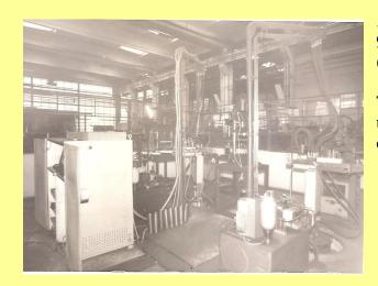
**9.6.** Command unit for production flexible cell (2 robots REH-03\* and 3 press machines) – 1985/1986, at Tehnofrig company Cluj-Napoca. This production cell was included in the technological production line of bottling machine exported in China.
