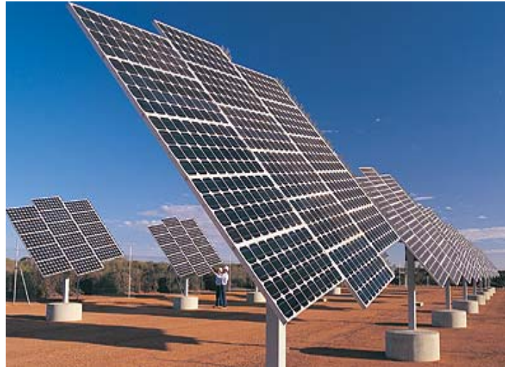
Figure 2. A photovoltaic pack with 2 axis tracker system
